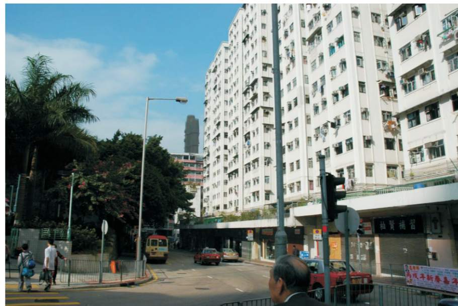
R3 Sai Wan Estate East Terrace, On Fat Building, Sincere Western House, Luen On Apartments, Luen Fat Apartments, Luen Hing Apartments, Luen Tak Apartments
