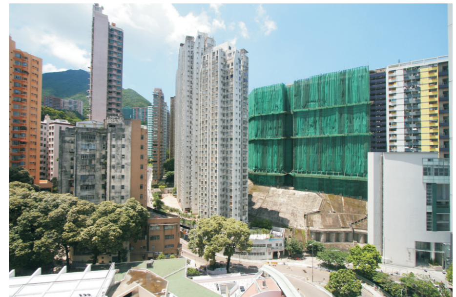
R4 Kwun Lung Lau, Smithfield Terrace, Pokfield Garden, Wai Wah Court, Poksmith Villa, Sun Fat Building, University Heights Tower
